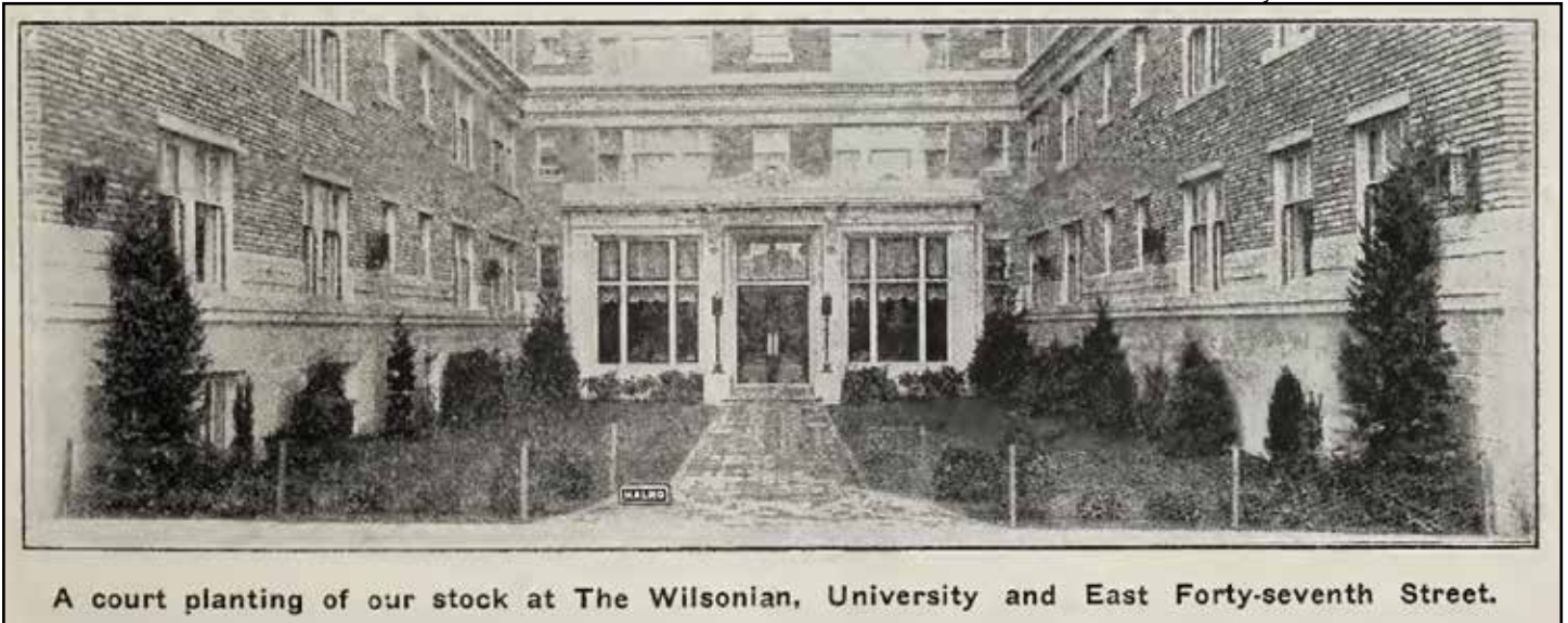
Figure 23 • The Wilsonian, 4700 University Way, Malmo & Co Spring 1924 Nursery Stock Planting Guide, (1923, architect and contractor: Frank Fowler, landscaper: Malmo & Company, extant)
